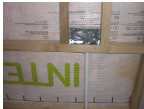
Above: A pro clima service grommet sealing a pipe penetration of the airtightness layer (left); A “service batten” on the inside of the INTELLO PLUS which reduces likely service penetrations of the membrane (middle); Overlaps of the Intelligent vapour check, INTELLO PLUS, sealed at critical junctions with pro clima airtight system proprietary seals (right)
